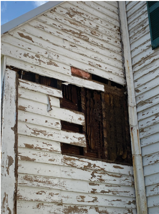
FIGURE 4.4 The wooden exterior cladding is removed revealing the honey bees, honey, and brood comb inside two voids created by wall studs.
